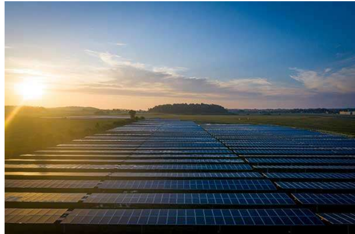
Solar energized at Morey Field. City purchased 0.5 MW of 5 MW “shared solar” system.
